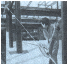
ABLE WRP used for steel alignment during erection.
